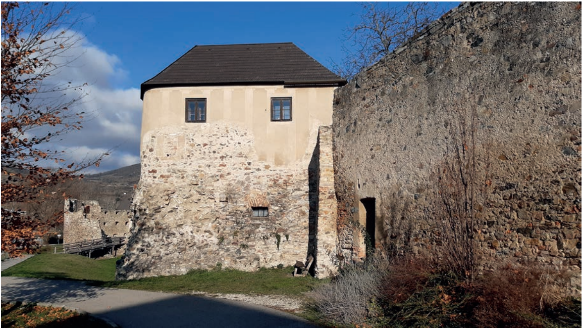
81. The curtain wall and the fan-shaped tower of the fort at Mautern is one of the best preserved examples of the Roman military architecture
