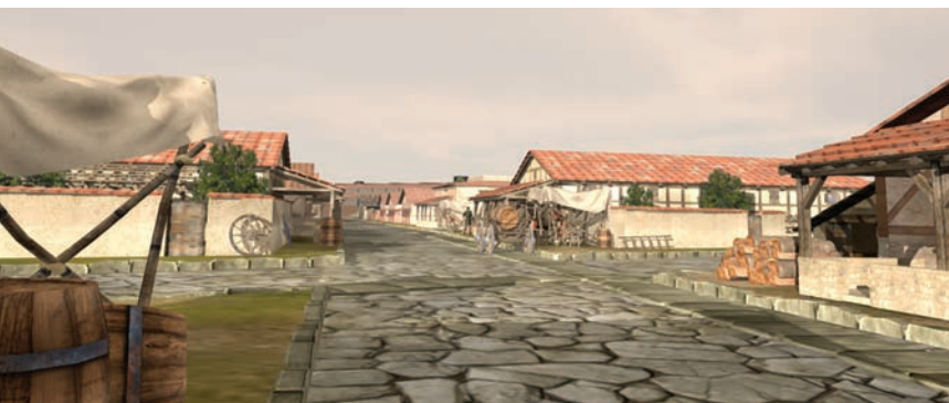
69. The Limes road connected the individual forts and main military installations. It was paved with stones close to the settlements, otherwise constructed with several layers of gravel
