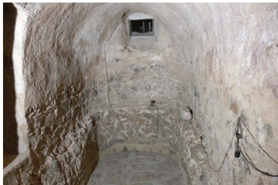
95. The remains of a U-shaped tower on the east front of the fort are preserved in the cellar at the Nikolaihof in Mautern
