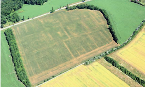
106. The irregular ground plan of the Carnuntum legionary fortress can still be clearly seen from the air today
