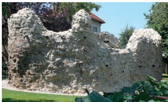
128. Fan-shaped corner-tower in Zeiselmauer after conservation
