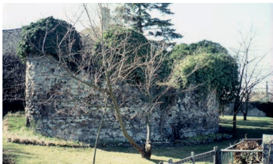
127. Fan-shaped corner tower in the fort of Zeiselmauer before the restauration
